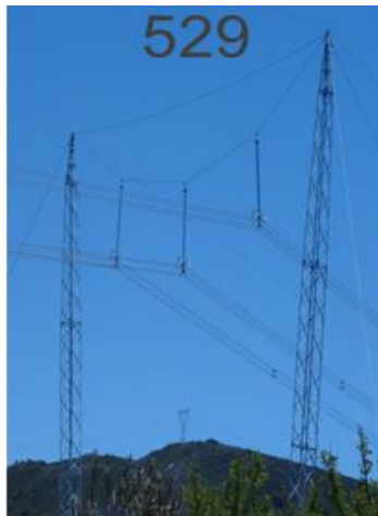
529a: Cross-Rope Suspension Towers
